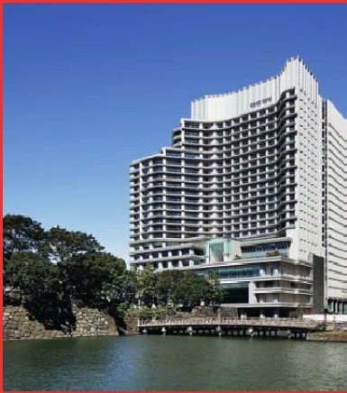
▲ The first spa is located on the fifth floor of the new US$1.2bn Palace Tokyo Hotel that reopened in May
